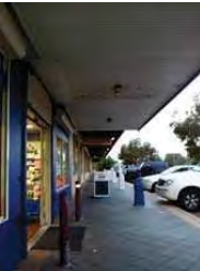
Inconsistent type, location, colour and maintenance of bollards. Exposed light fittings, poor lux readings, inconsistent lighting types and some are not in use. Signs of new and old graffiti along store face.
