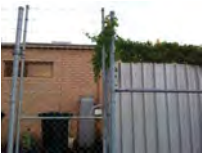
Fencing cross bar, overgrown vegetation and lack of visibility (sheet fencing) promote a potential climbing point.
