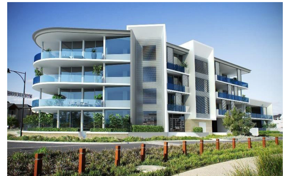
Photograph 33. A combination of open, solid and adjustable elements facilitate optimised airflow
