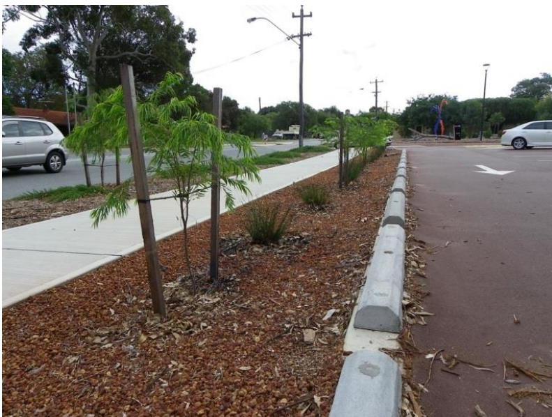
WSUD allows stormwater to drain from a car park into a bed of native plants at the Carawatha Park, Willagee
