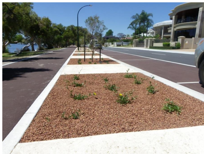
The streetscape upgrades on The Esplanade, Brentwood have removed kerbs to allow stormwater to drain into garden beds
