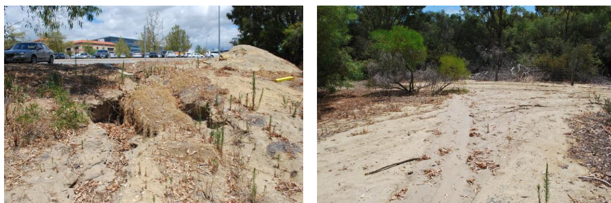
Figure 10: Stormwater runoff from hospital carpark causing erosion
