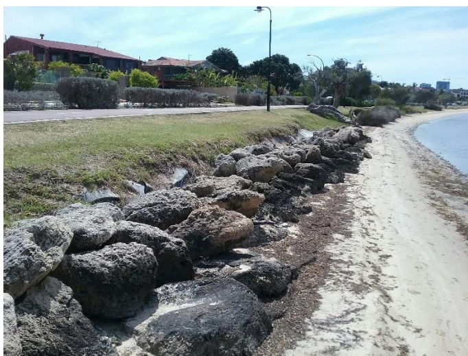
Figure 6-2 Slumping of rock revetment wall, Esplanade (Queens Rd), Mt Pleasant
