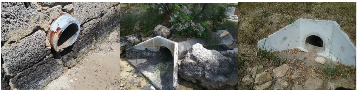
Figure 3-3 Drainage Outlets (2019)
