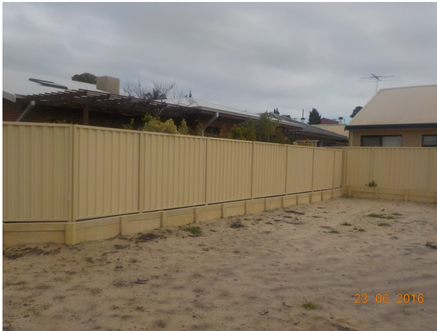
Figure 2. Existing retaining wall and boundary fence.
