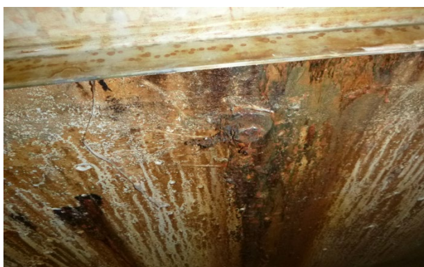
Concrete deterioration in the Gutters
