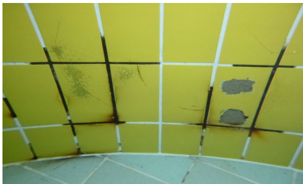
Rust Staining on the tiles
