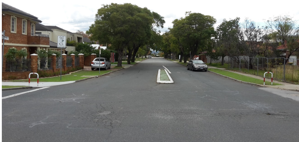
Figure 6. Northbound view along Forbes Road in the vicinity of subject site
