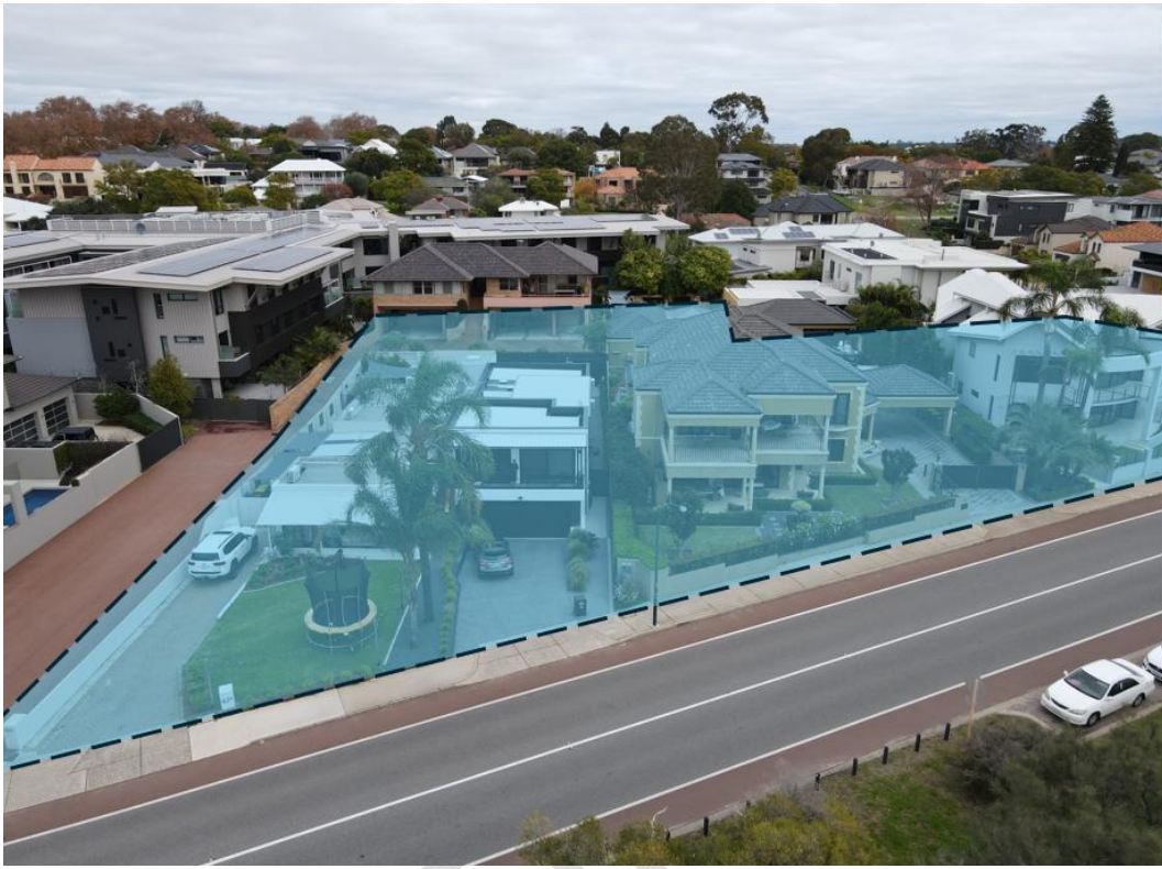
Figure 14 - View Looking West at Subject Land Comprising of 5 Residences Across 4,642sqm (combined)
