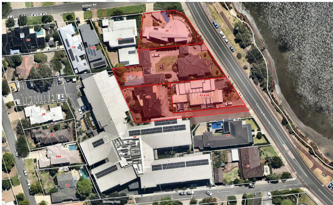
Figure 11- Aerial View of Subject Land Highlighted in Red
