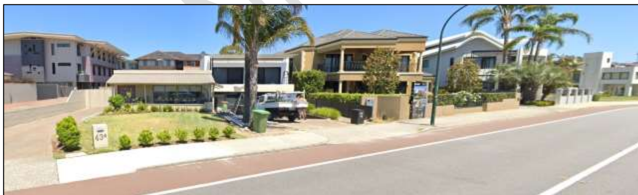
Figure 2: Streetscape view north-west along Canning Beach Road (subject lots)
