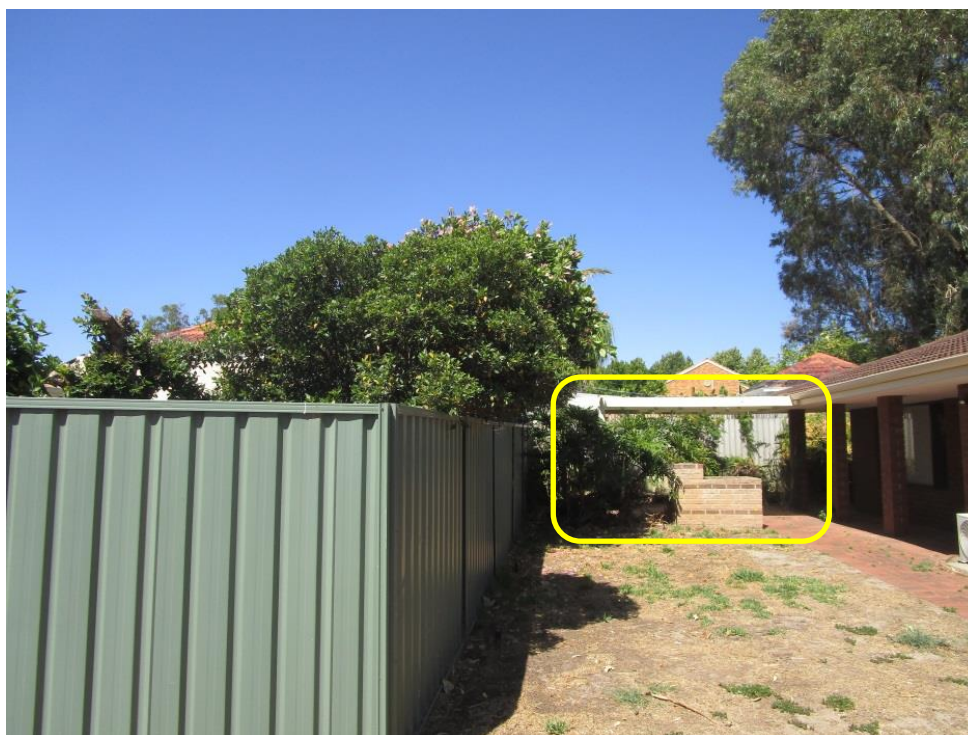
Figure 5: View of the boundary between the subject site and 2/13 Wren Street. The rear property's OLA is identified in yellow
