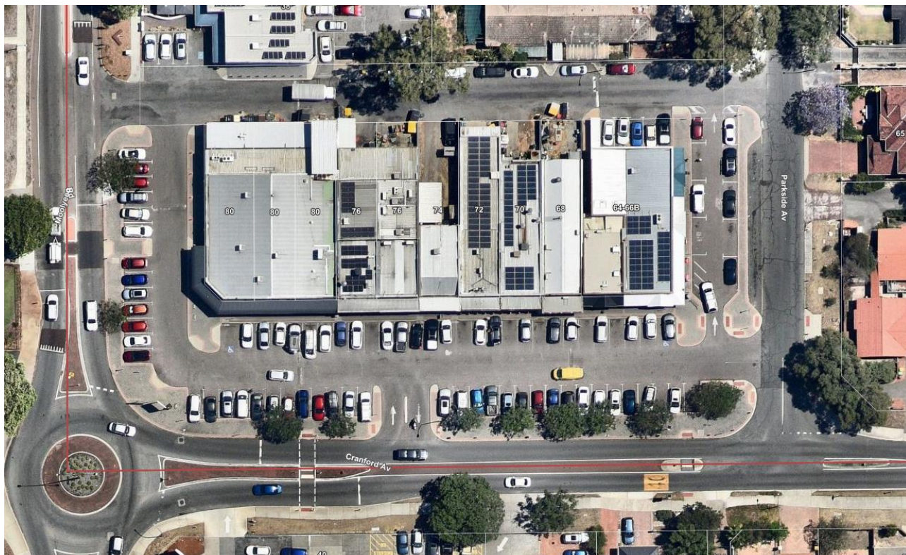
Aerial image of Brentwood Village Shopping Centre
