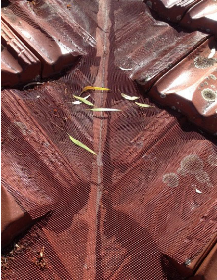
Mesh Installation: Picture Taken Mar 2016
