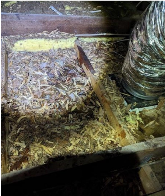
Roof Cavity: Picture Taken June 2023
