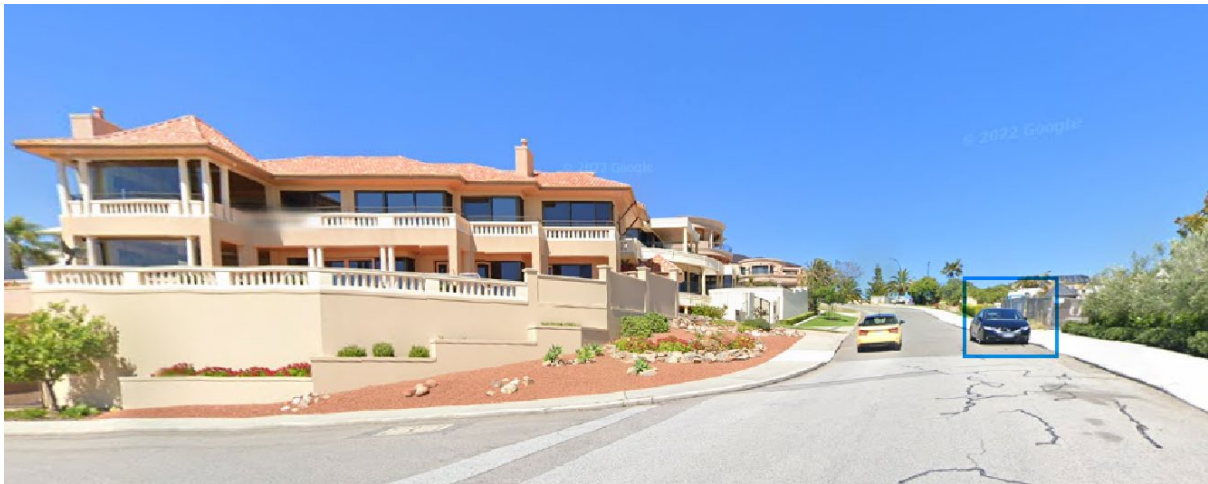
Figure 3: Street View Image of 1 Fraser Road.
