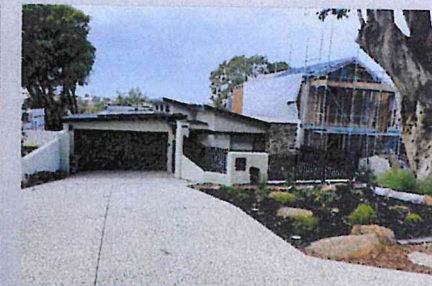
10E build completion
