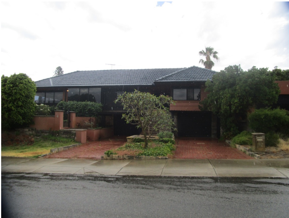
Figure 7: View of the middle portion of the existing home as viewed from Dee Rd
