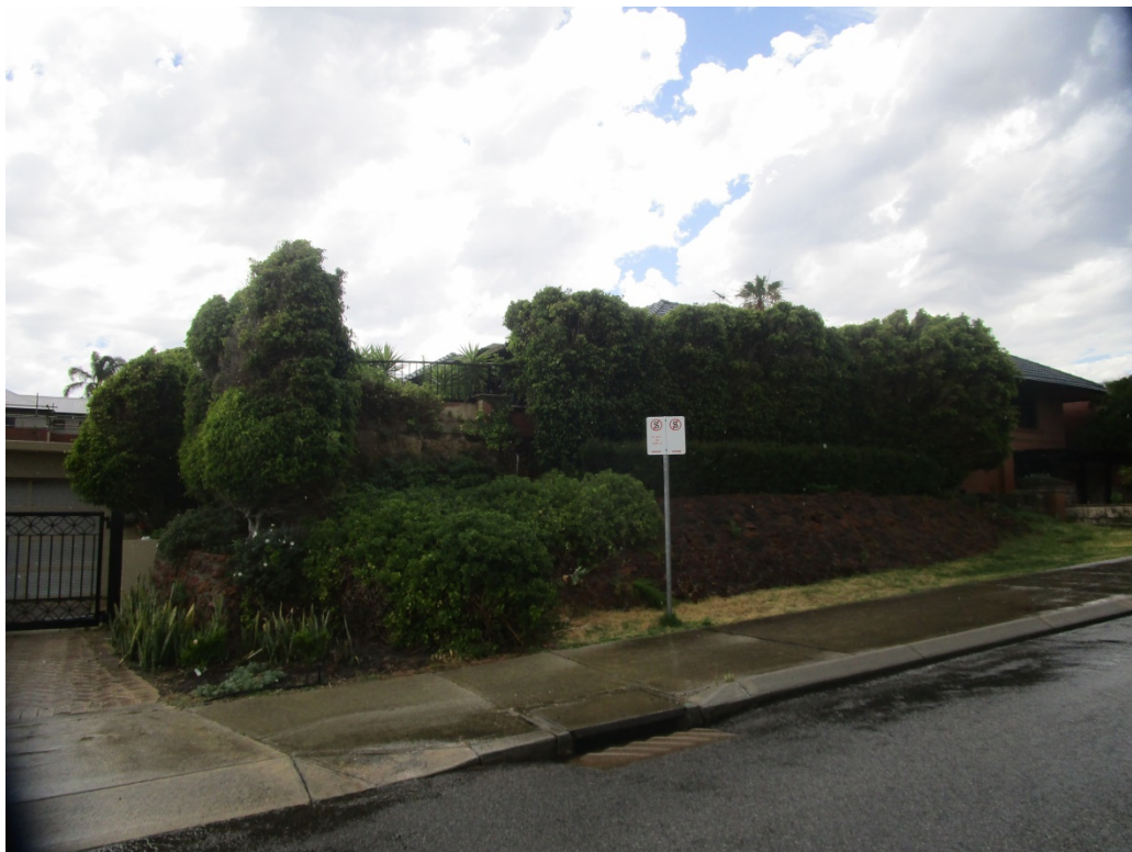
Figure 9: Area of retaining and fill which is to be removed within the verge and front setback on the western boundary
