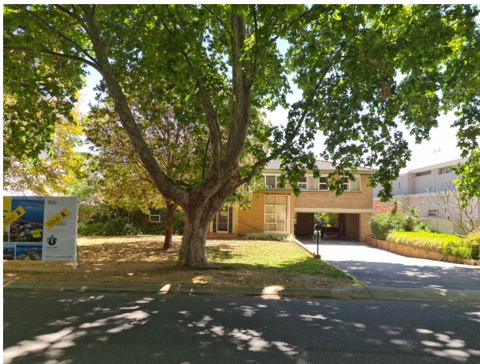
Figure 10: View north of the existing dwelling from Tweeddale Road. The tree seen in the foreground is to be retained
