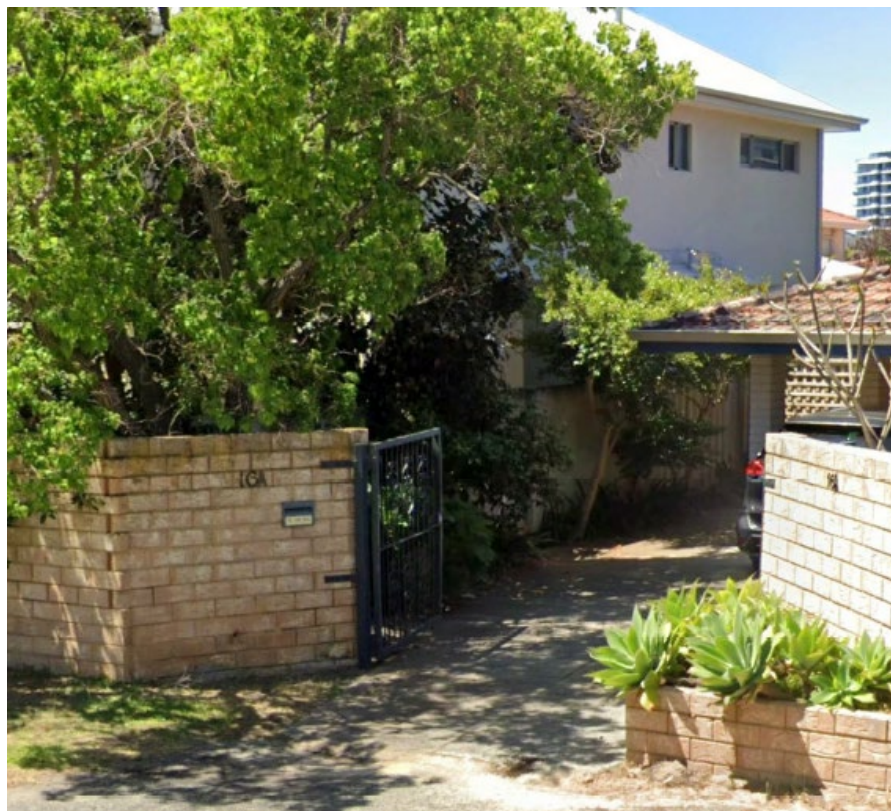
FIGURE 3.2 – R2 HIGH LEVEL WINDOWS
