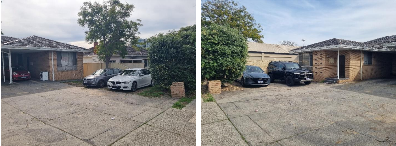
EXISTING PARKING, FRONT 862 CANNING HIGHWAY
