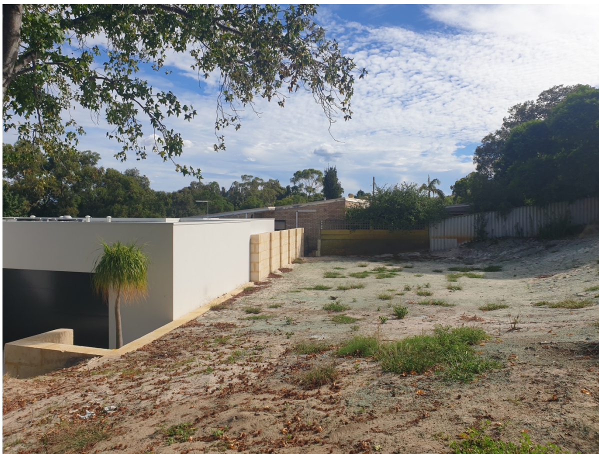
Figure 3: Southern boundary depicting existing boundary wall, retaining walls and dividing fence of adjoining property.
