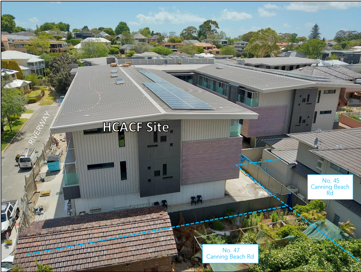
Figure 3 – View of HCACF looking west from No. 47 Canning Beach Rd (17 December 2021)
