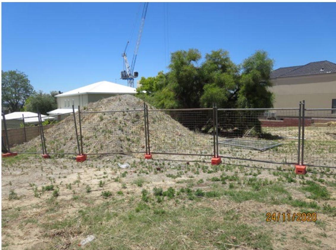
Photograph 1: Unauthorised material on site, November 2020
