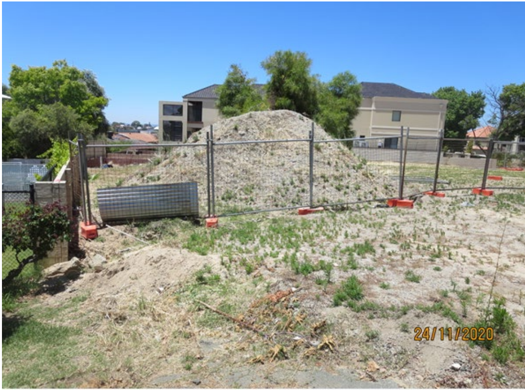
Photograph 2: Unauthorized material on site, November 2020
