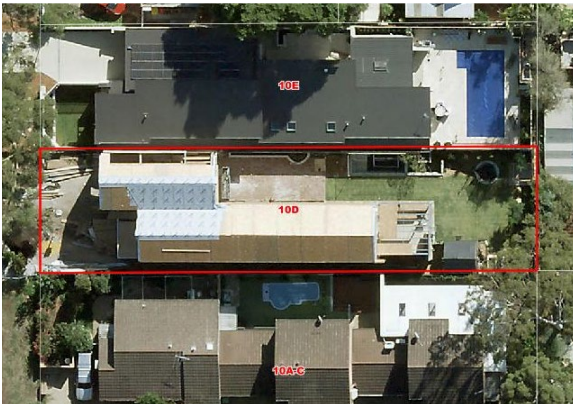
Figure 1: Aerial photography of subject site (No. 10D Birdwood Circus, Bicton)
