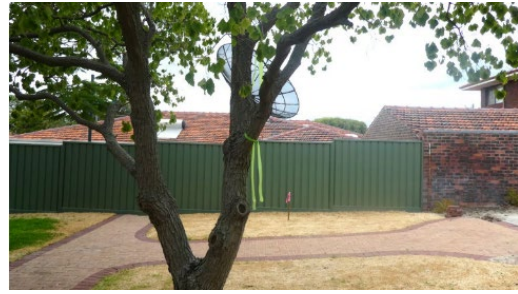
Figure 7: Existing dividing fencing on the southern elevation (Source: Applicant Site Photo)
