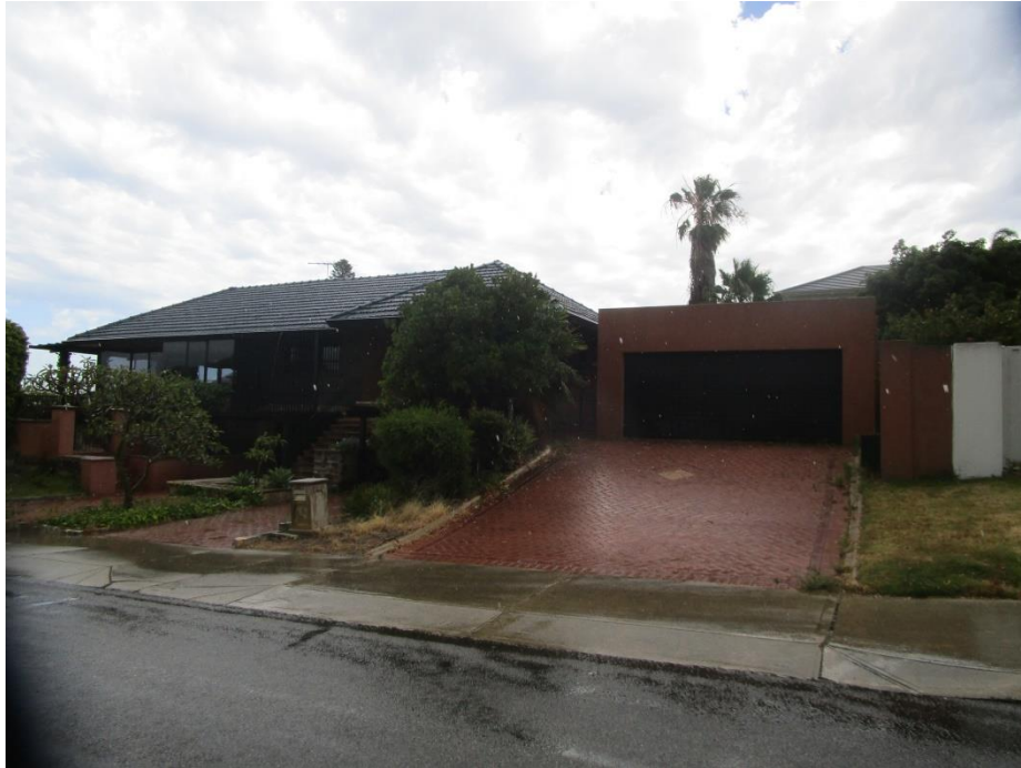
Figure 8: Existing driveway serving above ground garage on the eastern boundary
