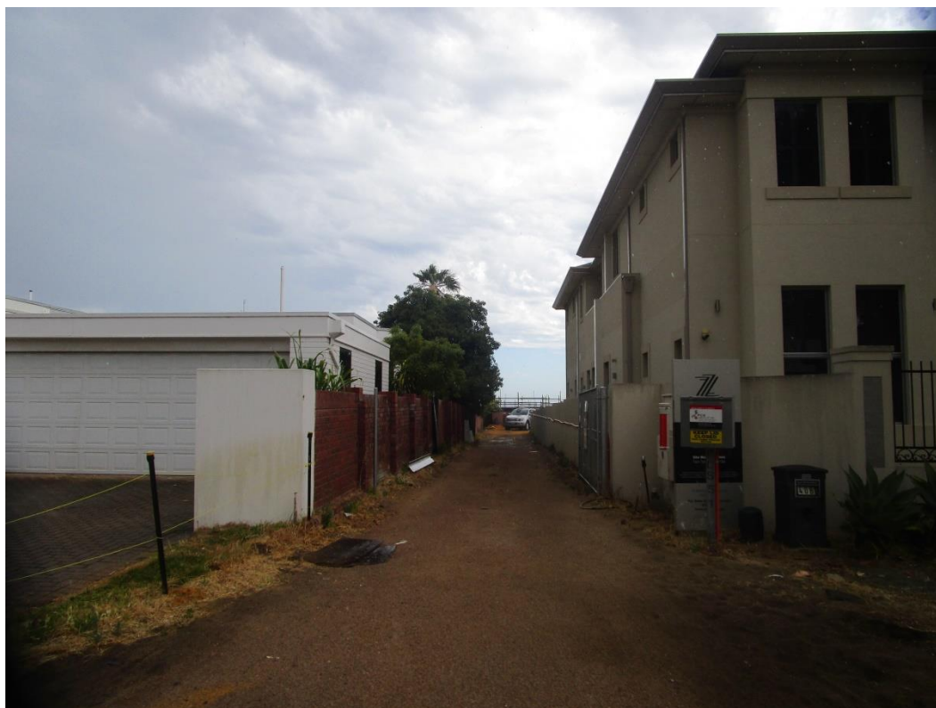
Figure 10: Access leg servicing the rear neighbour at 40B Fraser Rd. this access leg will alleviate the bulk impact from the proposed development
