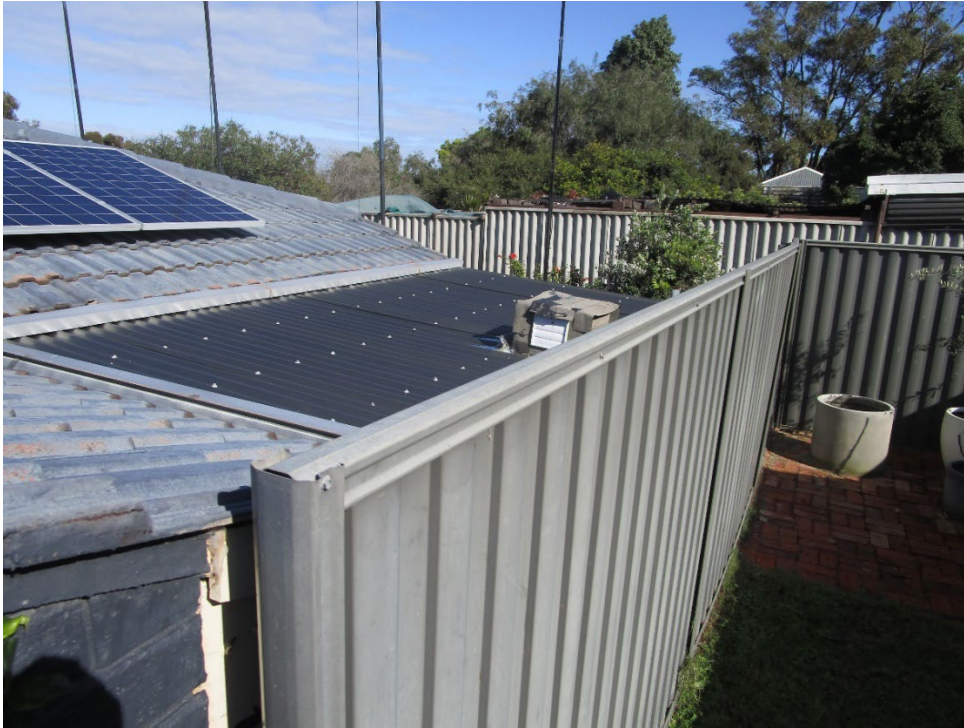
Figure 5 – Taken from the subject site into the southern property (15A Redwood Court northern boundary). COV falls onto the roof of the carport.
