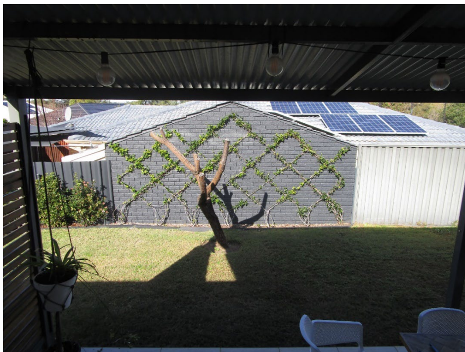
Figure 4 – A view of the southern boundary of the subject site. This photograph has been taken at the proposed FFL of the future alfresco and living room.
