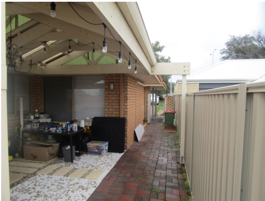
Figure 3: Photo showing height of No.26 McGillivray Gardens covered outdoor living area and eaves which are to be of a similar height of the proposed patio columns.
