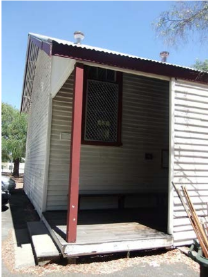
School – northeast corner.
