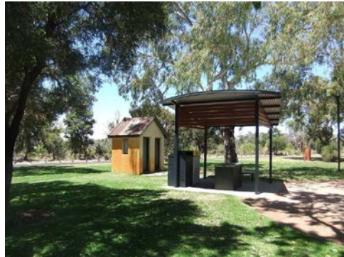
Small toilet block.
