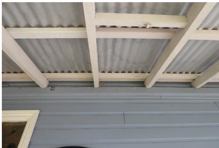
Original veranah wall plate
