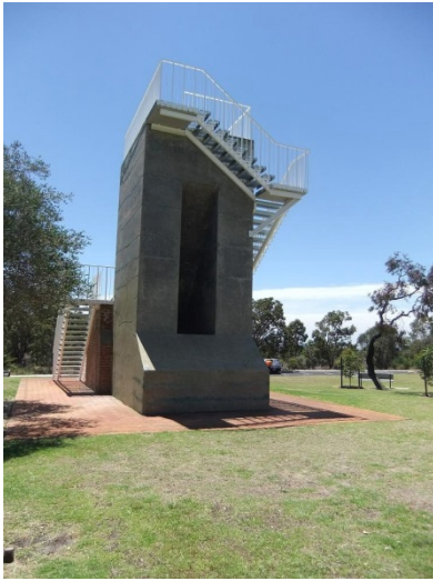
North anchor block.
