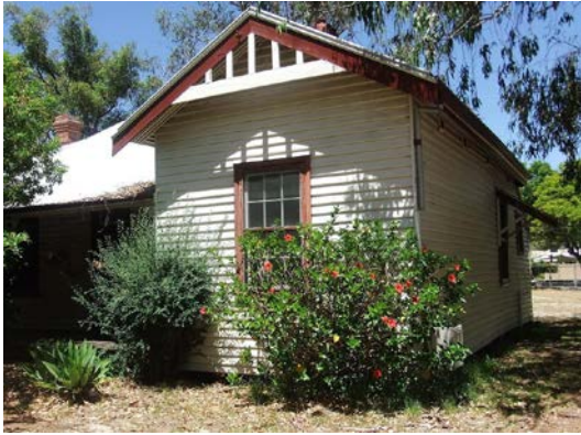
Teacher's House – north elevation.
