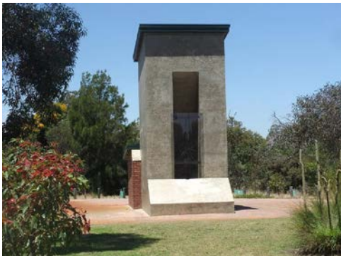
South anchor block.
