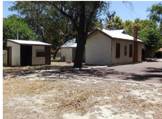
View looking north to Teacher's House and outbuilding.
