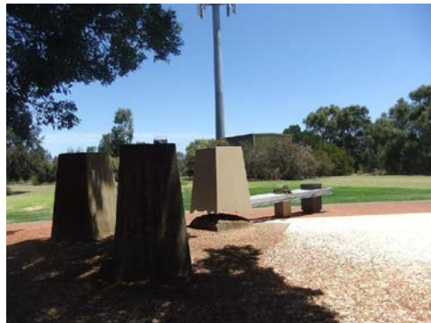
Guy anchor blocks for aerial mast.
