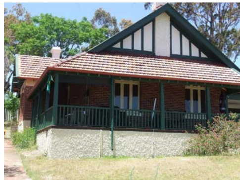
No. 8 Hickey Street – former staff house.
