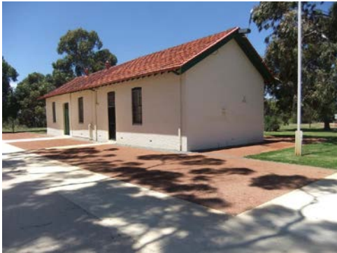
Capitol Radio and toilets – former Store.
