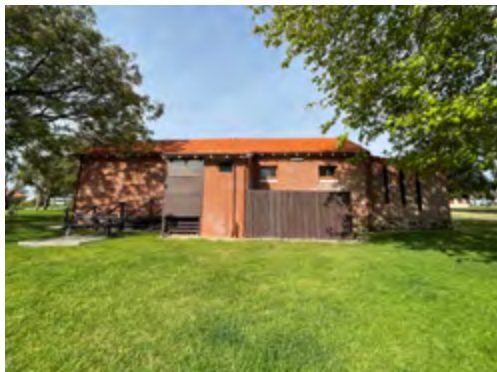
Building exterior (west)
