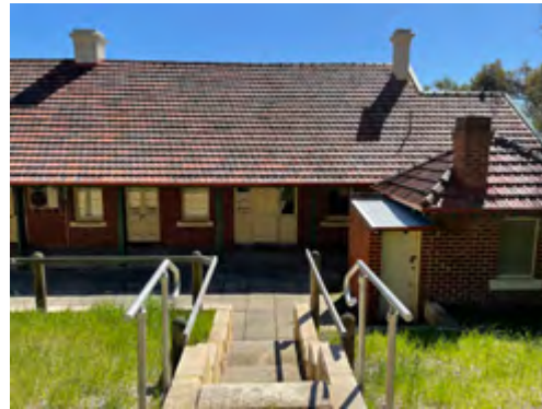
Rear of cottage #6
