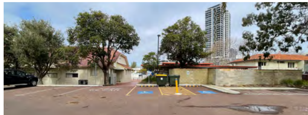
Canning Bridge Library exterior (north)
