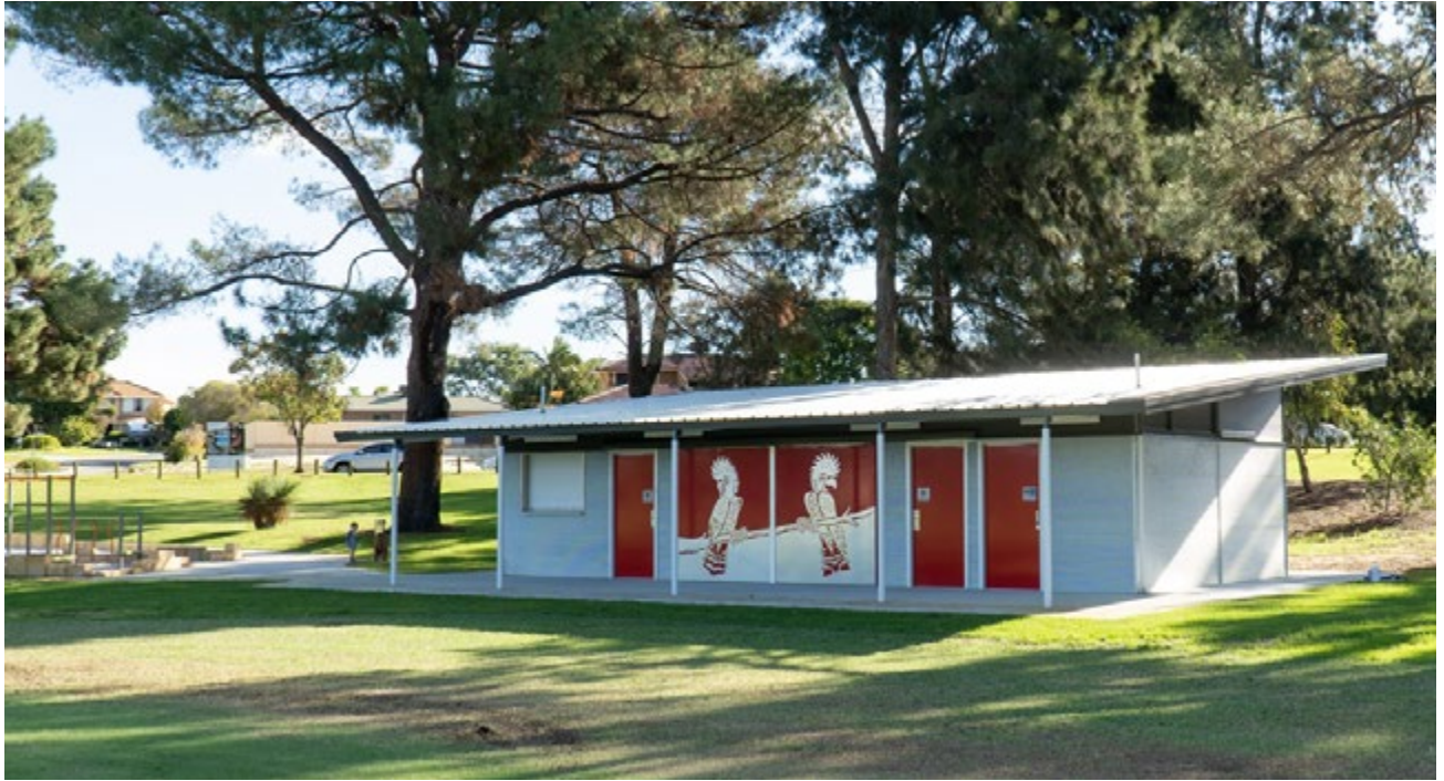
This year we started and completed construction of a new amenity building at Bert Jeffrey Reserve.
