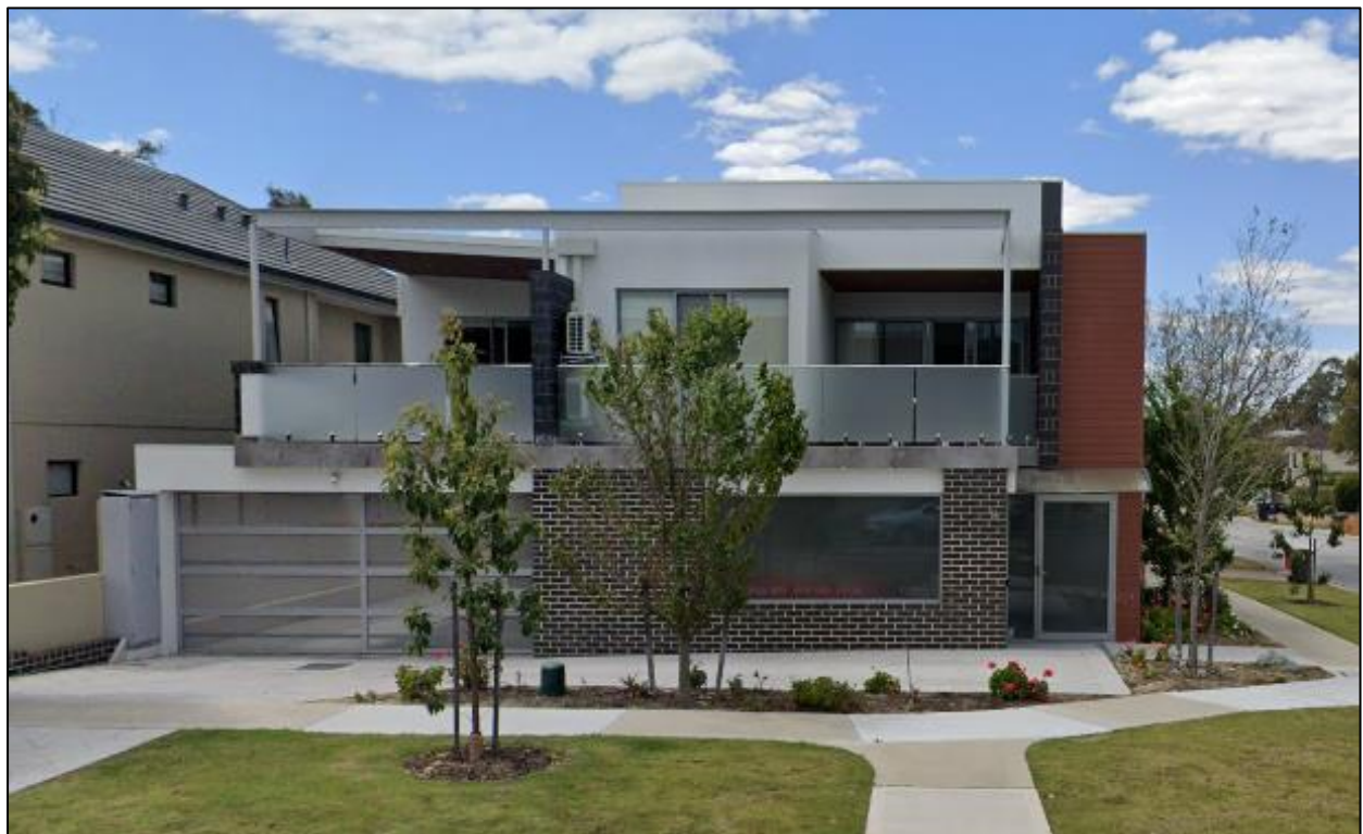
Figure 17 – Yokine 'apartment house' example
