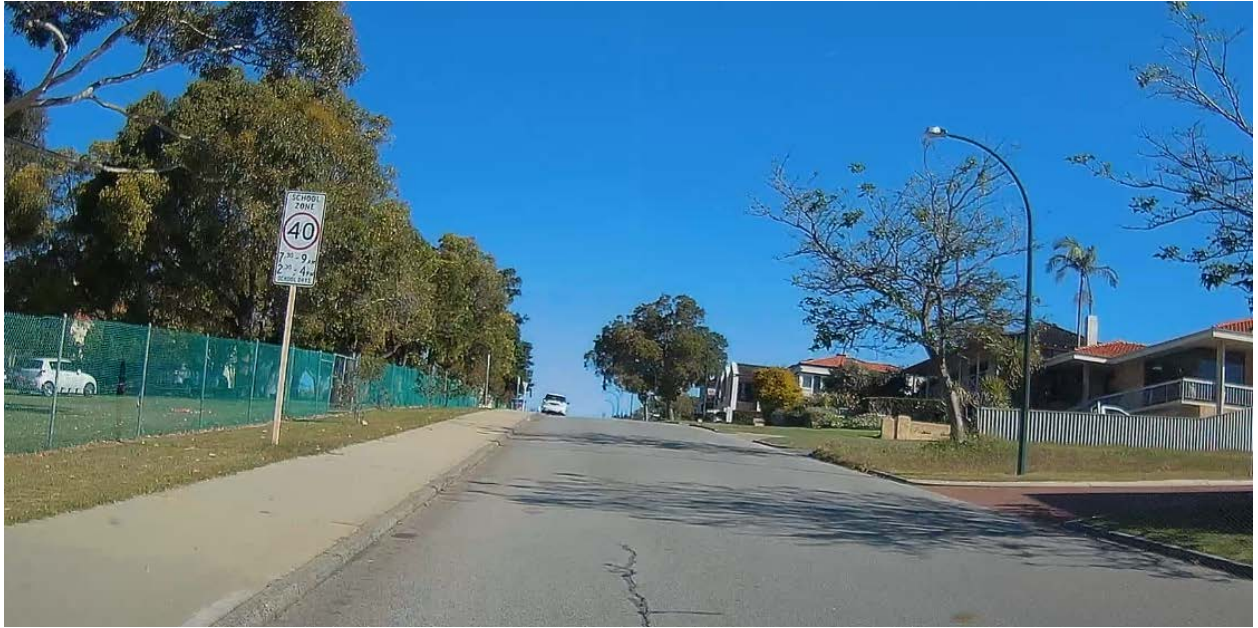
Figure 2 – Moreing Road, north of Stoneham Road
