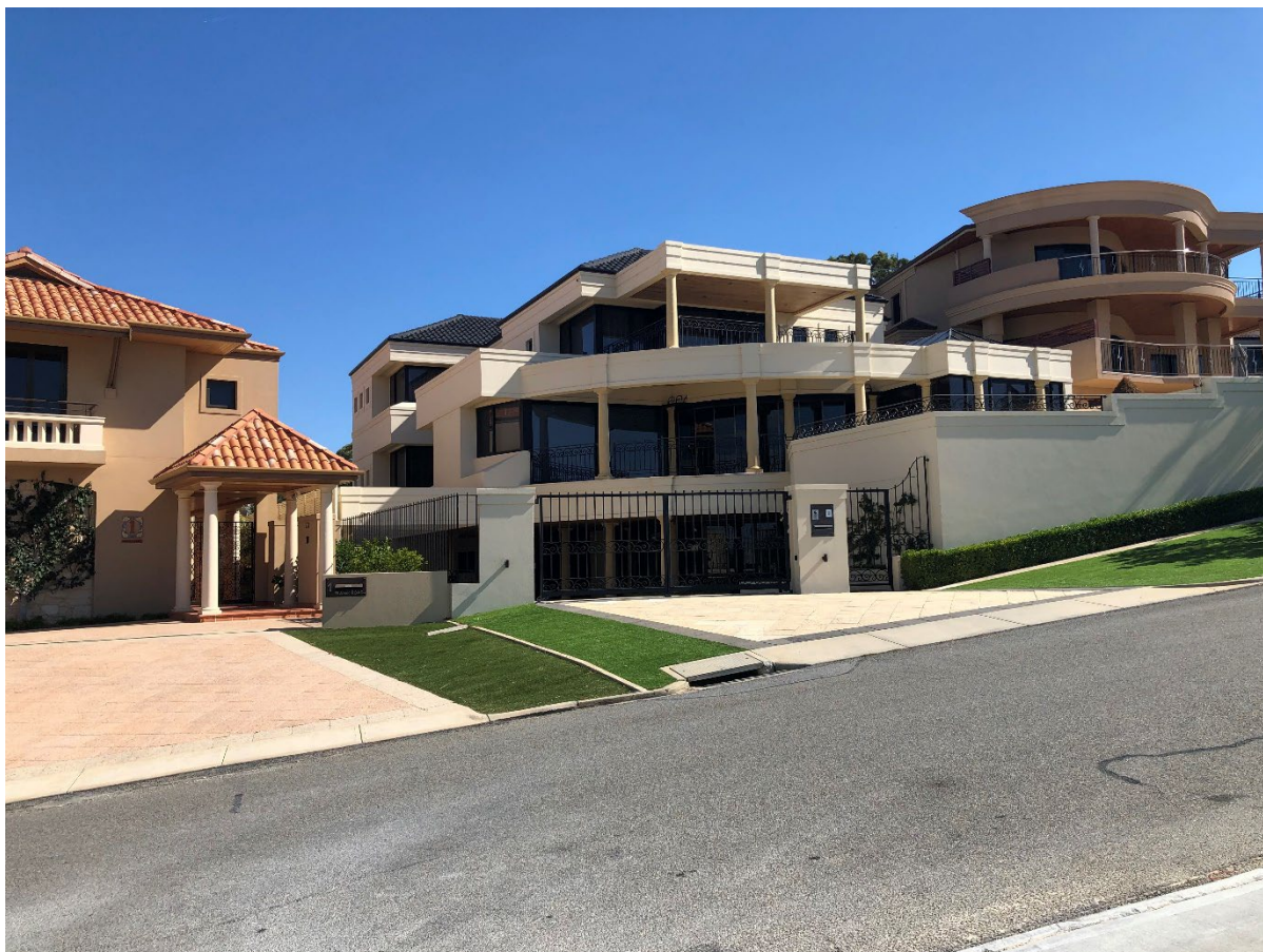
Figure 2: Site Photo Showing Ground Floor & Upper Floor Balconies at No.3 Fraser Road
