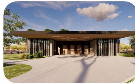
Charging hub at Matilda Bay
