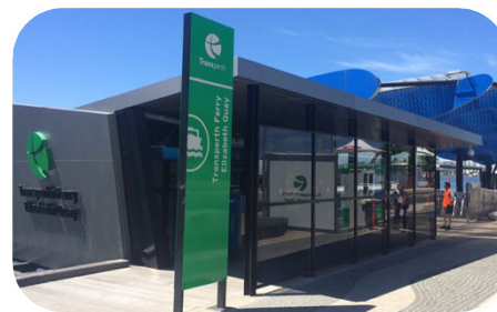
Elizabeth Quay jetty upgrades
