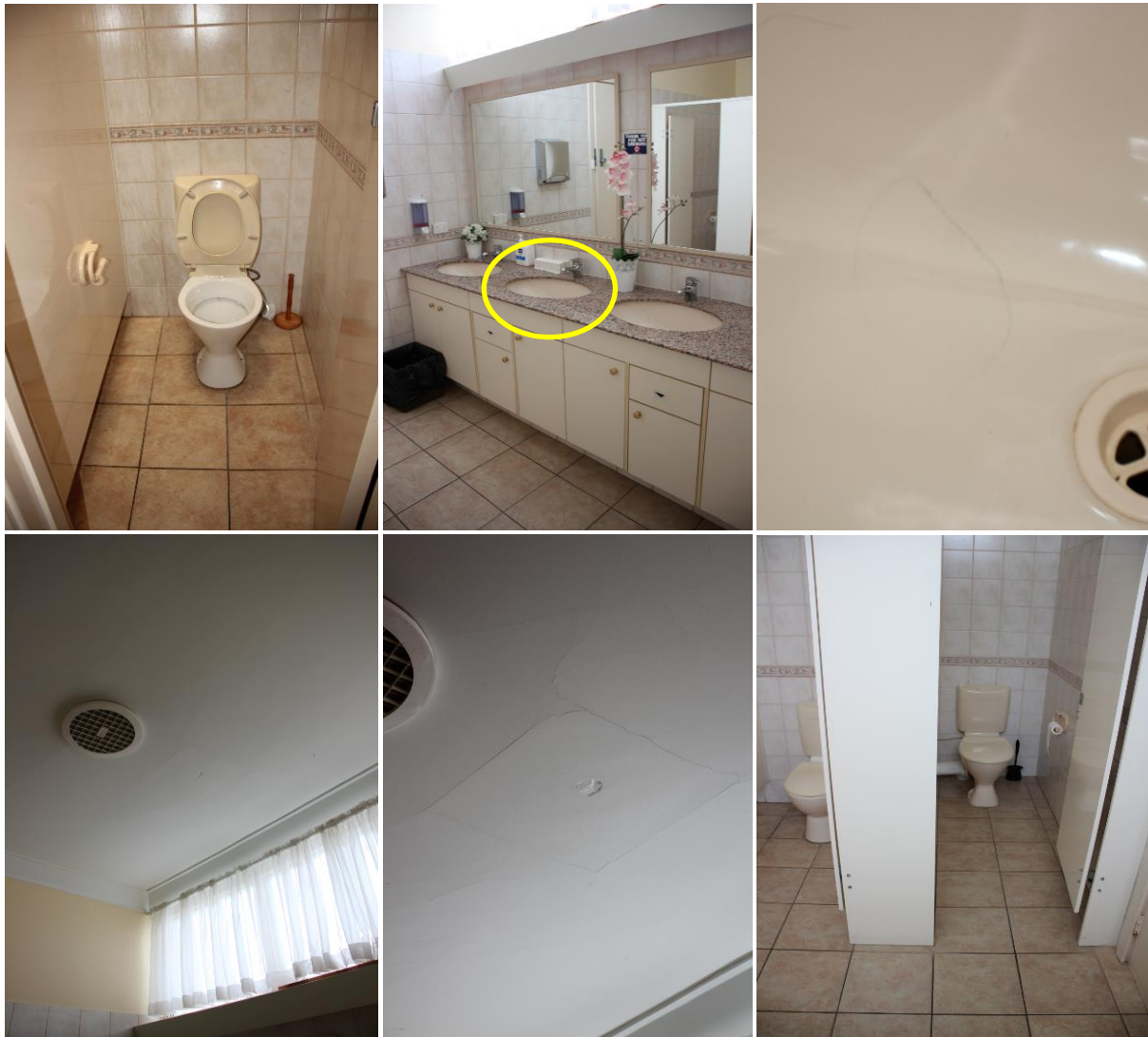
Figure 27: Photo 120, 121, 122, 123, 124 & 125 – Ladies bathroom
