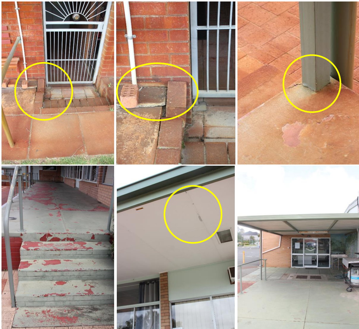
Figure 5: Photo 27, 28, 29, 30, 31 & 32 – Verandah and eaves lining
