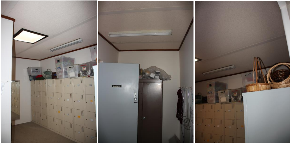
Figure 26: Photo 117, 118 & 119 – Ladies locker room
