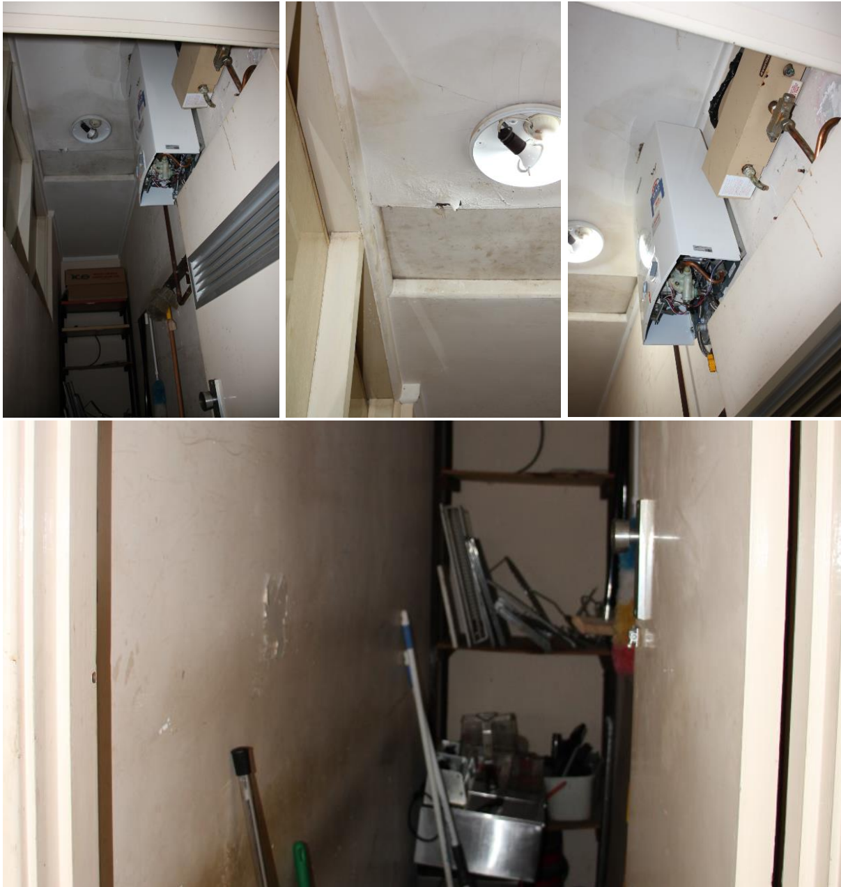
Figure 24: Photo 106, 107, 108 & 109 – Service duct
