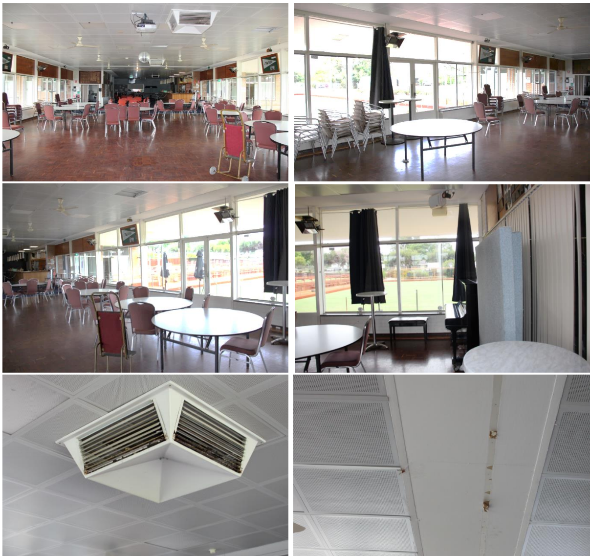
Figure 9: Photo 45, 46, 47, 48, 49 & 50 – Main hall
