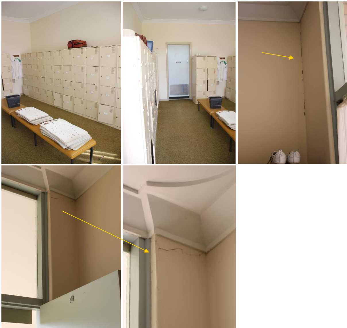
Figure 18: Photo 81, 82, 83, 84 & 85 – Men's changeroom
