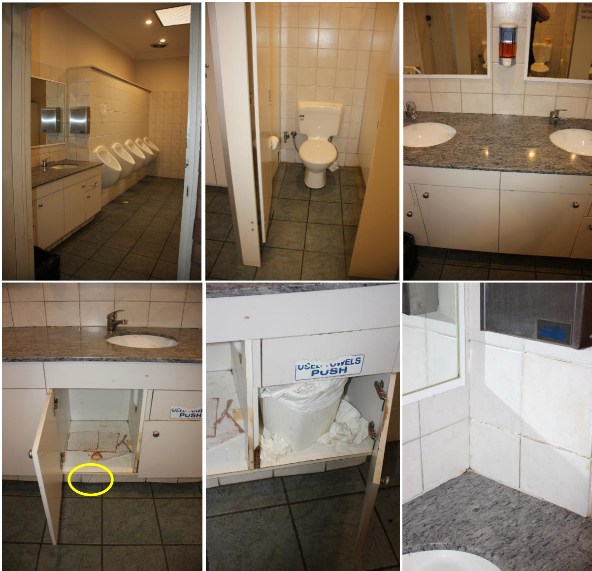
Figure 17: Photo 75, 76, 77, 78, 79 & 80 – Men's bathroom
