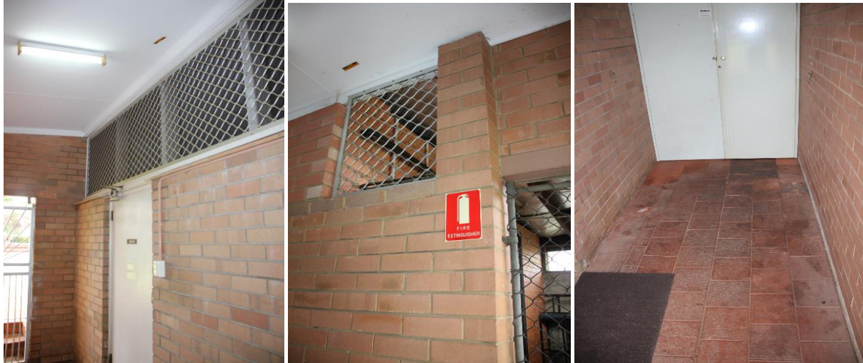
Figure 15: Photo 69, 70 & 71 – Male toilets
