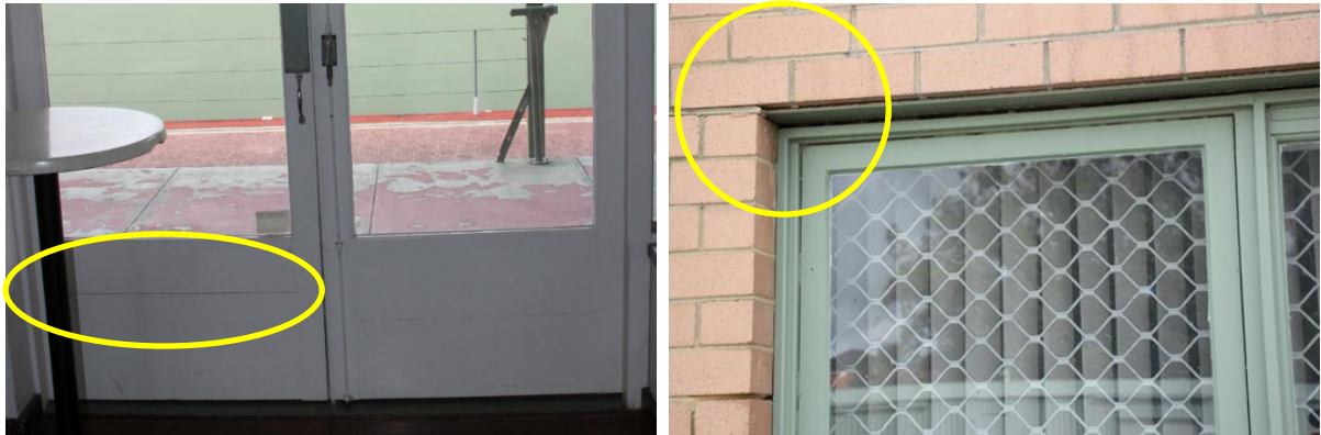
Figure 3: Photo 17, 18, 19, 20, 21, 22, 23 & 24 - Windows and doors
