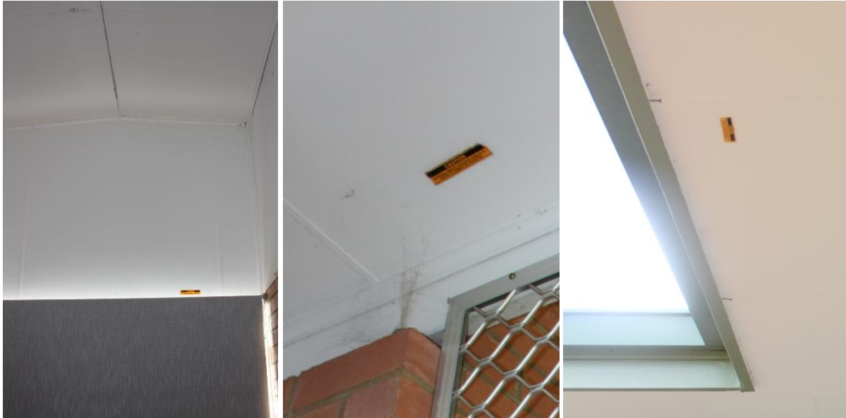
Figure 33: Photo 152, 153 & 154 – Asbestos
