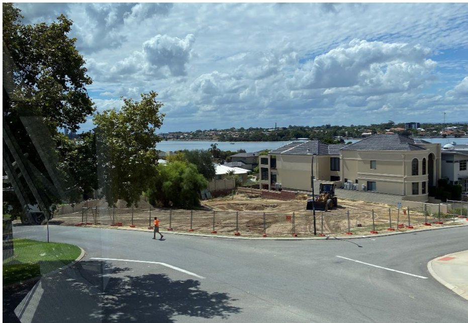
G) Photo_Unauthorised Fill_16 March 2020_12.30 PM 2-3 more (4 th , 5 th & 6 th ) mounds of sand added & levelled
