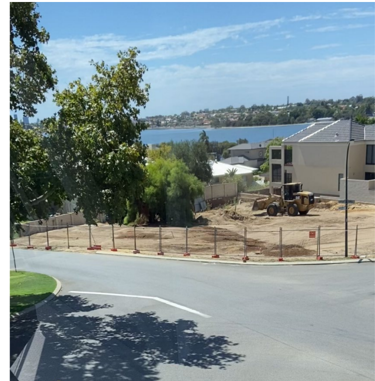
C) Video Still_Unauthorised Fill_13 March 2020 1rst sand mound levelled
