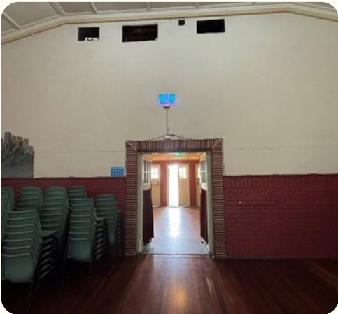
Figure 56 East wall of the hall showing face brick door architrave and dado (contemporary paint).
