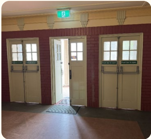
Figure 52 Entry lobby front doors.
