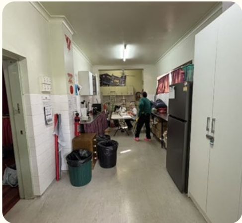
Figure 58 Kitchen wing located on the north.
