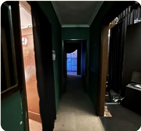
Figure 63 North hallway running alongside the stage.
