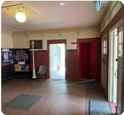
Figure 55 Overview of the entry lobby.
