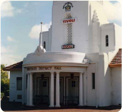
Figure 33 Frontage of the subject site, dated 1997.
