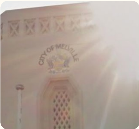
Figure 35 City of Melville branding prior to removal, dated October 2015.
