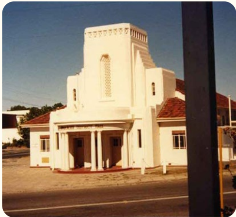
Figure 30 Frontage of the subject site, dated 1981.
