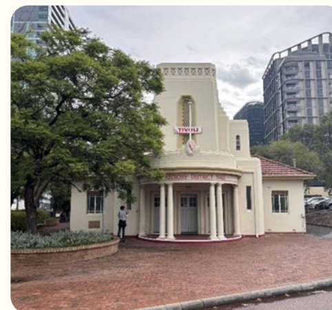
Figure 44 East elevation, principal entrance existing condition note Jacaranda trees to the south.
