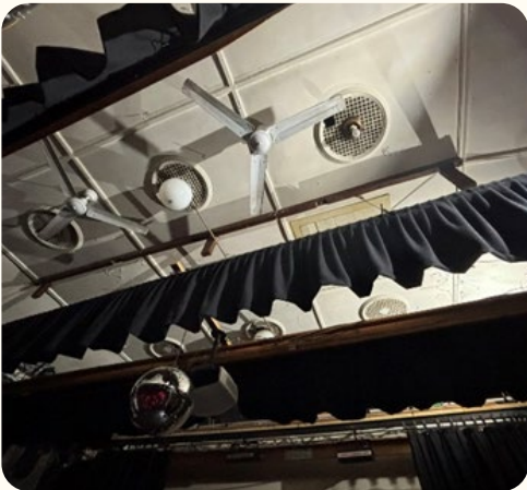
Figure 62 Strapped ceiling to the stage with circular roof ventilators.
