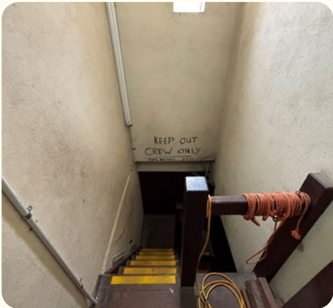
Figure 54 Timber stair to the bio box.
