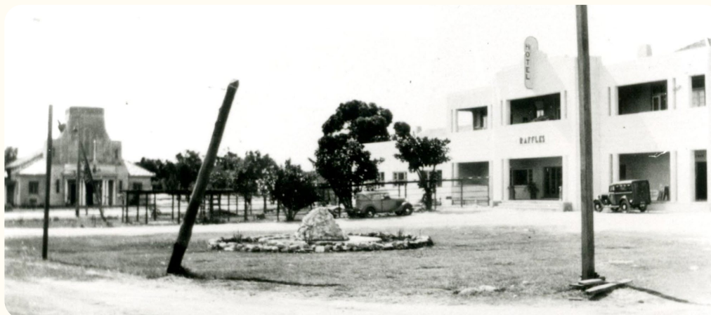
Figure 18 Raffles Hotel with the subject site to the left, dated 1939.
