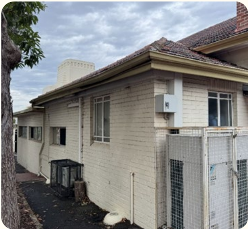
Figure 50 Extended kitchen block existing condition
