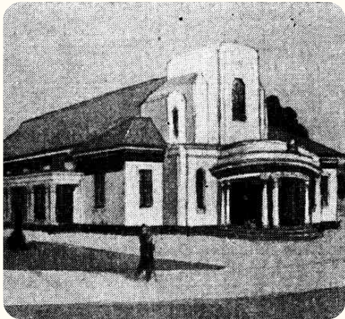
Figure 14 Illustration of Applecross District Hall after construction, c. 1937.
