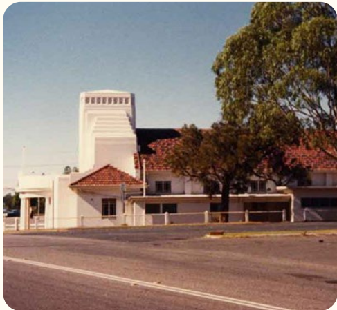
Figure 31 Frontage of the subject site, dated 1981.
