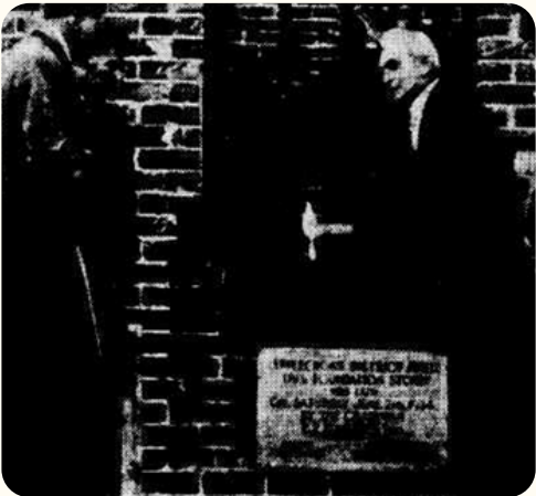
Figure 8 Chairman of the Melville Road Board (Mr E.F. Edwards) laying the foundation stone of the Applecross District Hall during construction, dated 1934.
