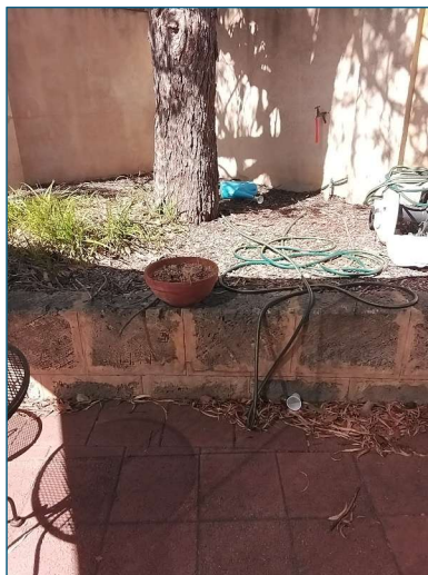
Image 24: Elevated location of Tree #12 and large walls in proximity
