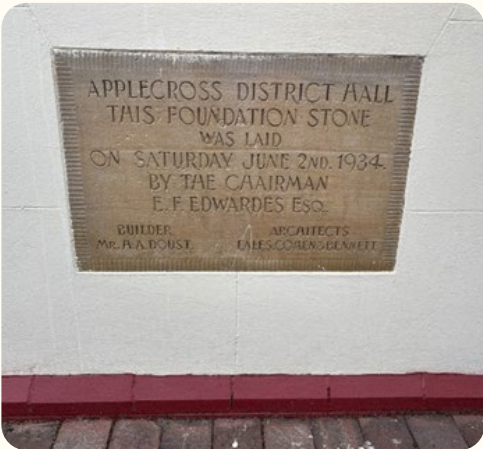
Figure 49 Foundation Stone located on the east elevation.
