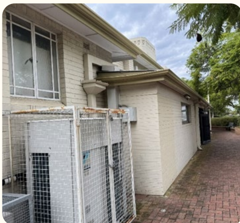
Figure 51 South elevation with altered original verandah.
