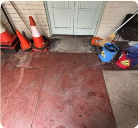
Figure 59 Flooring between the north storeroom and kitchen is presumed to be the concrete from the original colonnaded verandah.
