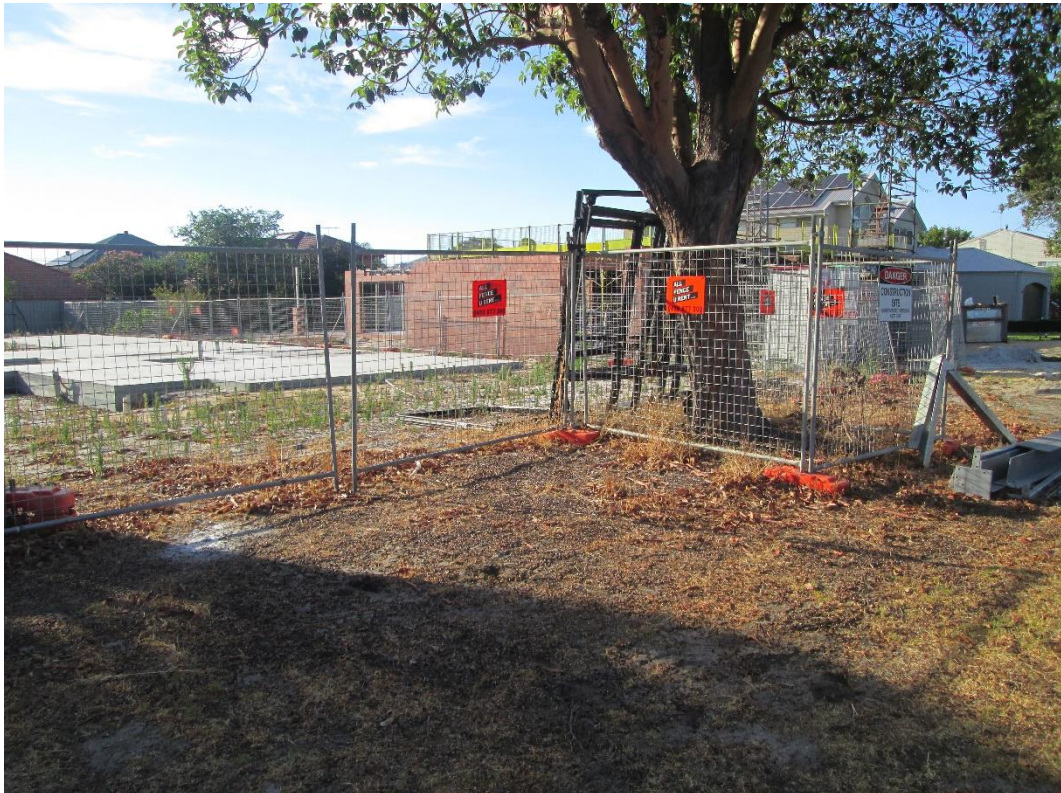
Figure 3 Displaying the tree in relation to the new construction works.
