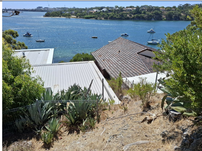
Figure 25. View West Over No.50 Blackwall Reach Parade.
