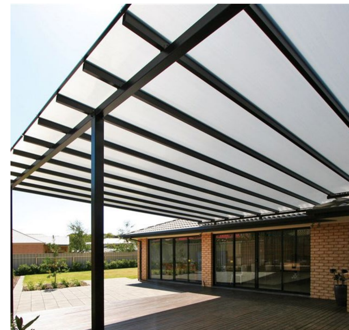
STEEL SHADE STRUCTURE WITH DANPALON PANELS
