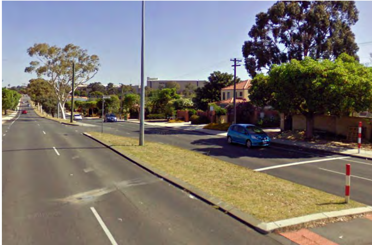
Figure 46 - Approach view of Garden City building and 'Myer' sign
