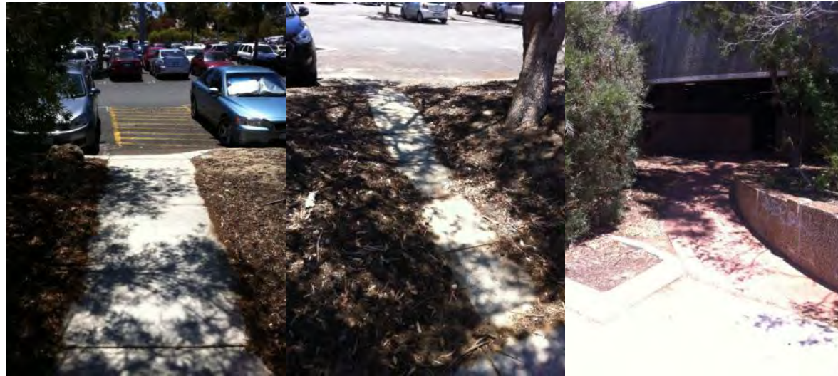
Figure 22: Poor access for people on foot
