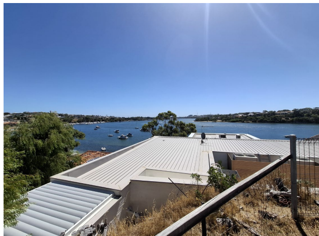
Figure 26. Additional View West Over No.50 Blackwall Reach Parade.
