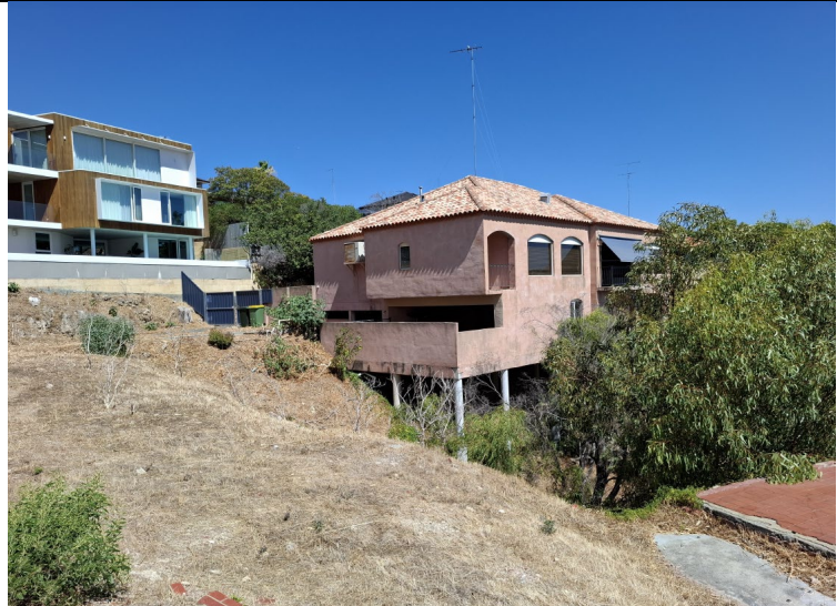
Figure 2. Shows Topography and steep Drop in Ground Level Below proposed Unit 2 Bed 1.
