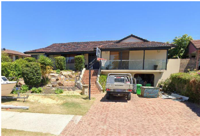
FRONT ELEVATION FROM LE SOUEF DRIVE
