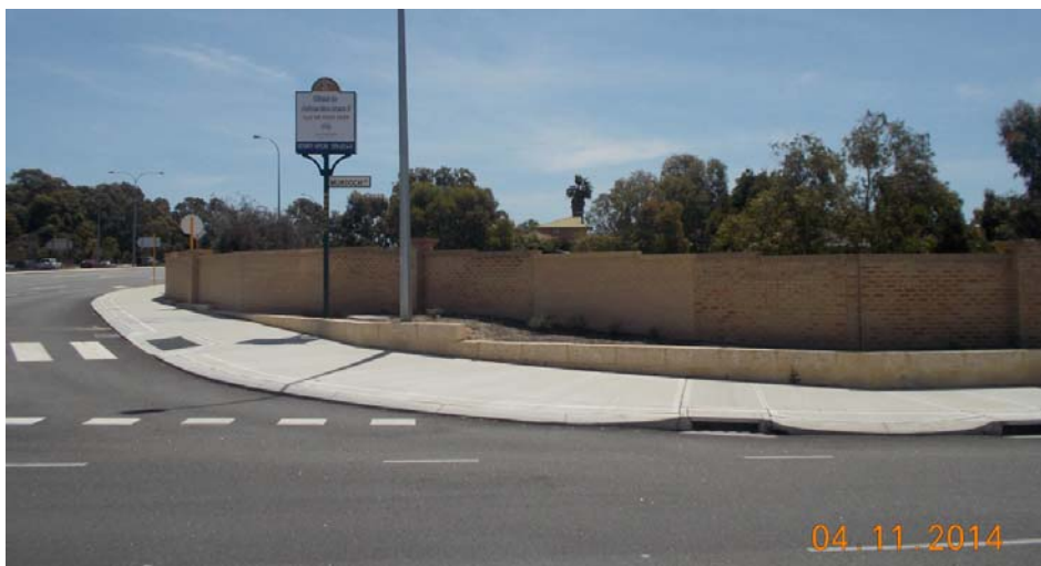
Image 1 – Affected portion of Reserve 39780 (sand behind retaining)
