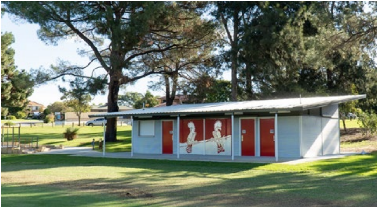
This year we started and completed construction of a new amenity building at Bert Jeffrey Reserve.
