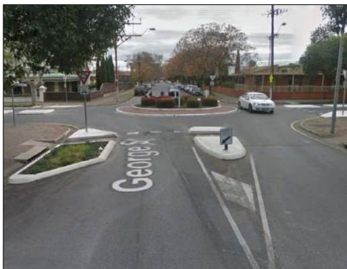
Figure 5-2: Radial Roundabout (George Street/Beulah Road, Norwood, SA)
