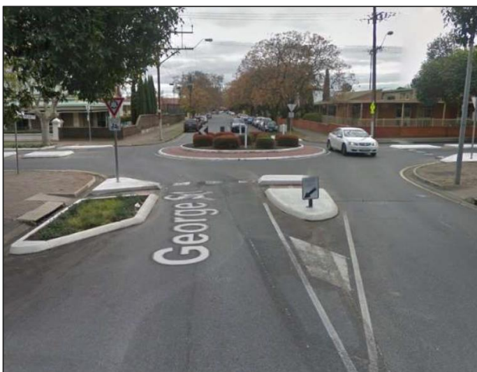
Figure 5-2: Radial Roundabout (George Street/Beulah Road, Norwood, SA)
