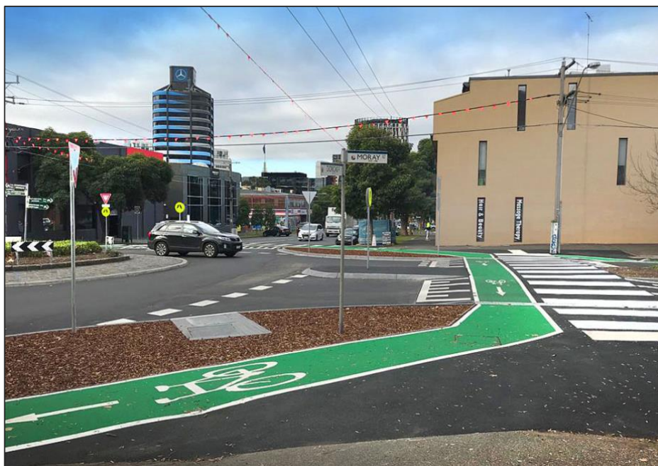
Figure 5-3: Roundabout Priority Crossing Points Set Back from the Entry (Moray Street/Dorcas Steet, Melbourne)
