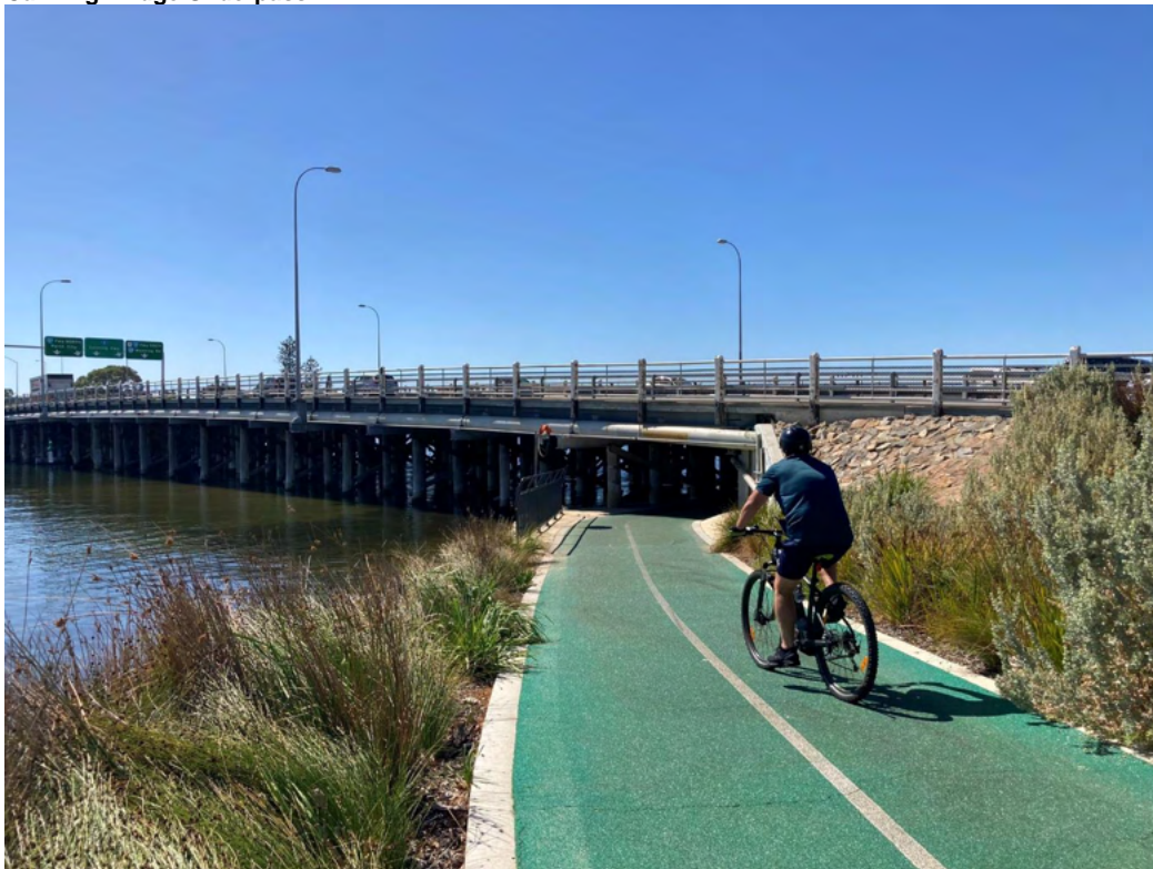
Foreshore Path Connecting with Dee Road
