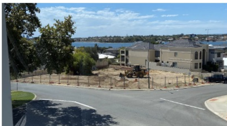
D) Photo_Unauthorised Fill_14 March 2020_8 AM Raised levels & tyre marks
