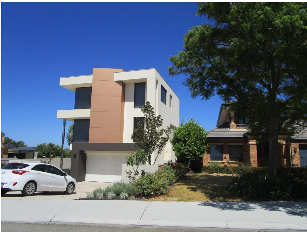
Figure 10: View of the neighbouring property at 14B Fraser Road.
