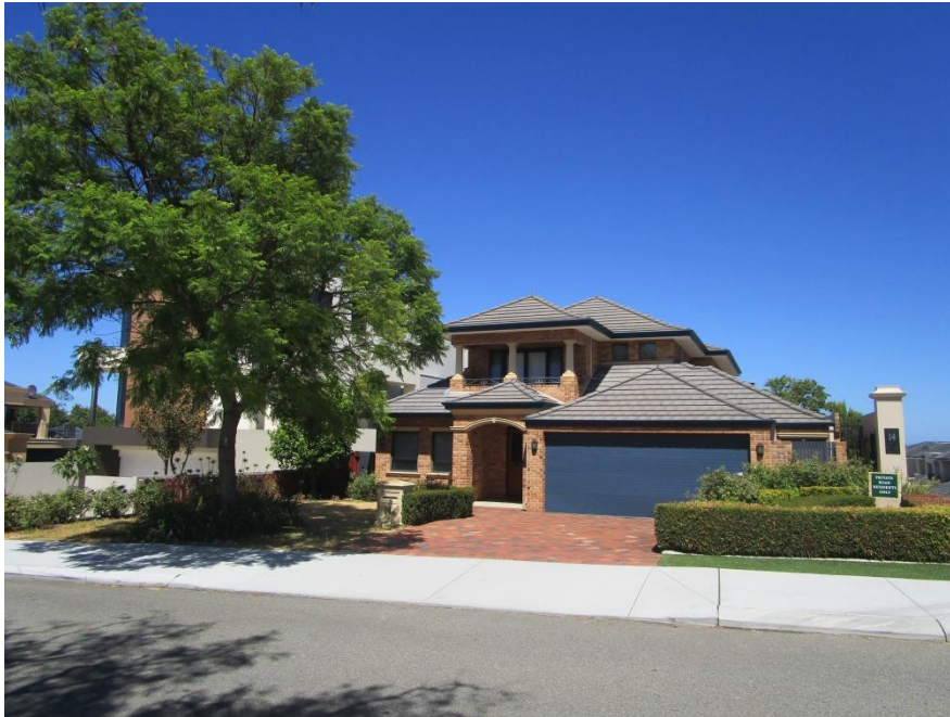
Figure 9: View of the existing two storey home from Fraser Road. This home is to be demolished.
