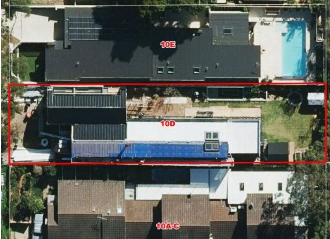
Figure 1: Aerial photograph of subject site (No. 10D Birdwood Circus, Bicton)
