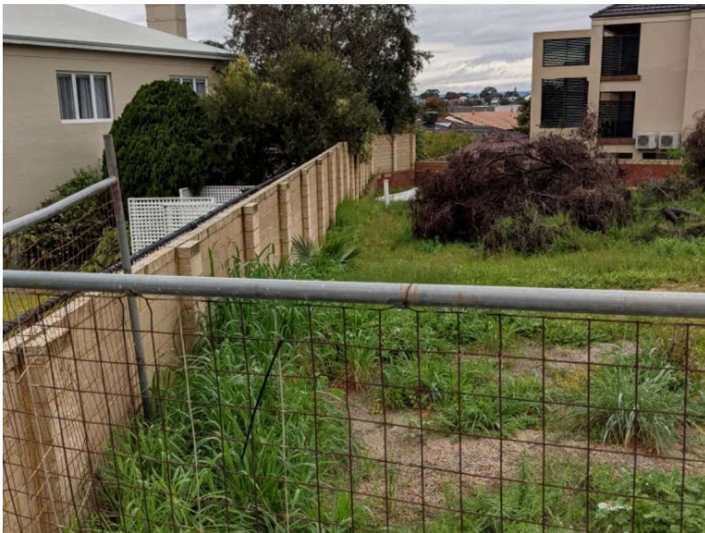
Photograph 6: 18 Tweeddale Road retaining walls in north east corner
