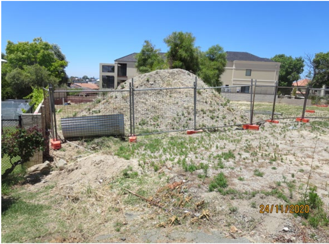
Photograph 2: Unauthorized material on site, November 2020
