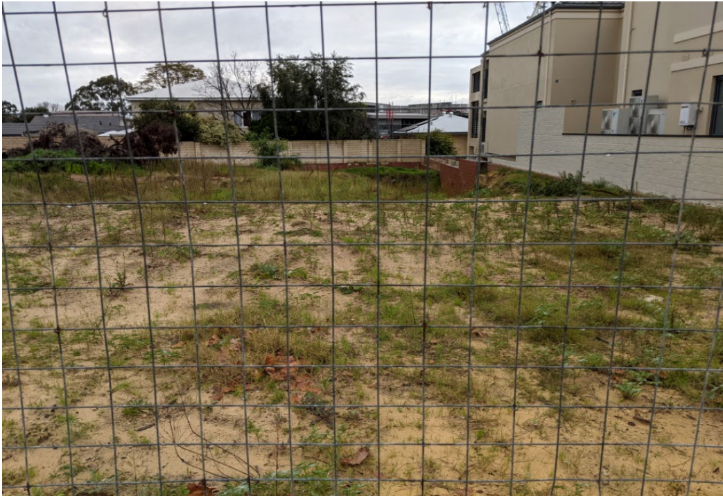
Photograph 5: 18 Tweeddale Road retaining walls to north and east side.
