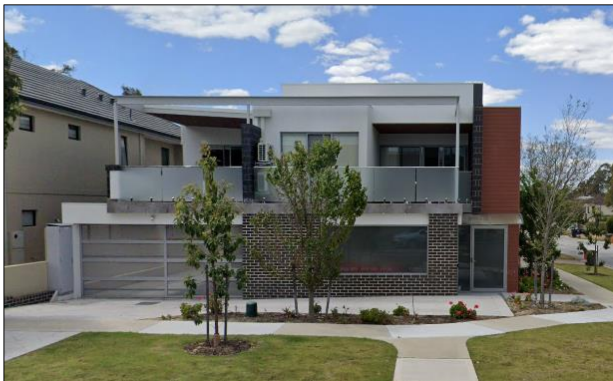
Figure 16 – Yokine ‘apartment house’ example
